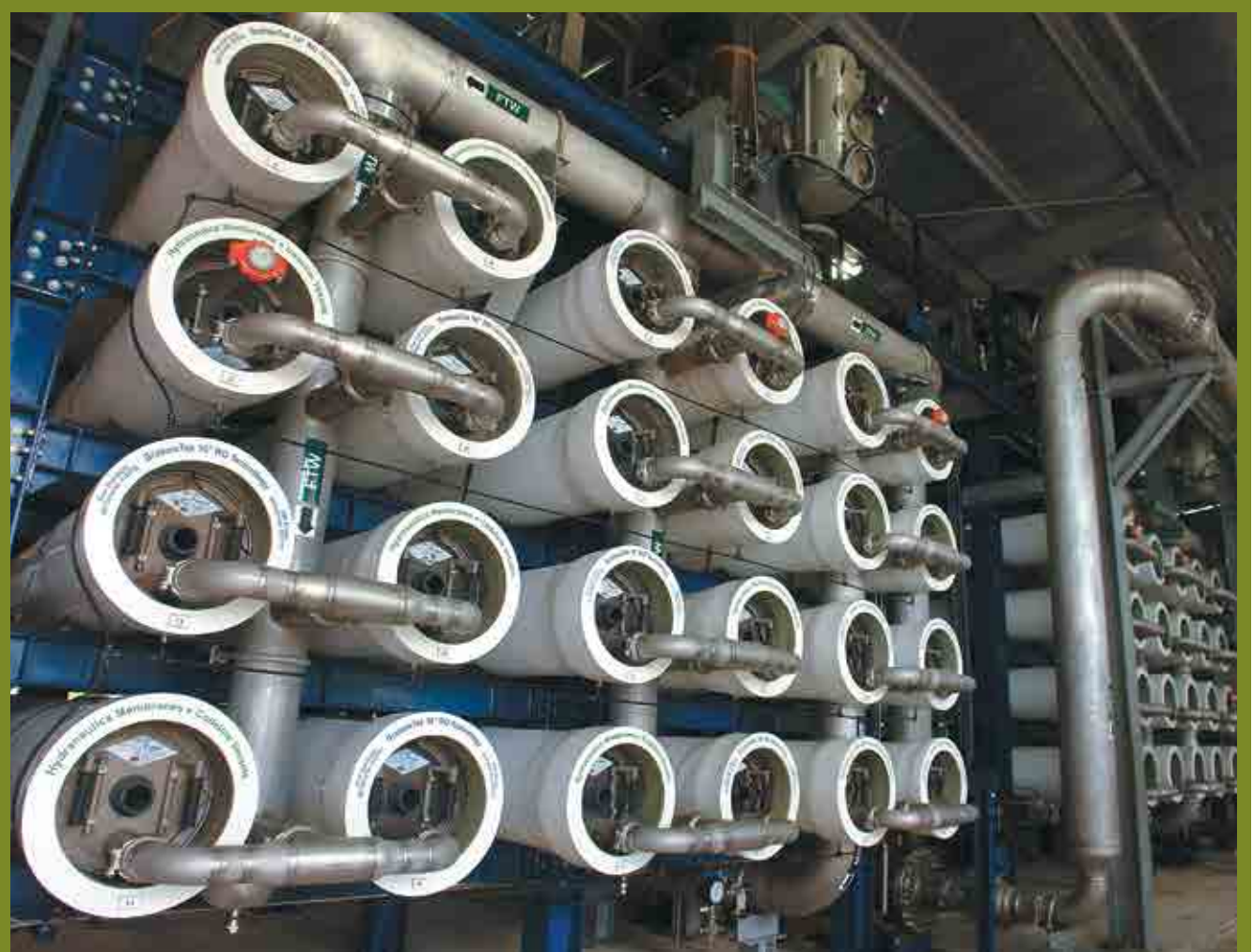
YTL PowerSeraya's Desalination Plant
