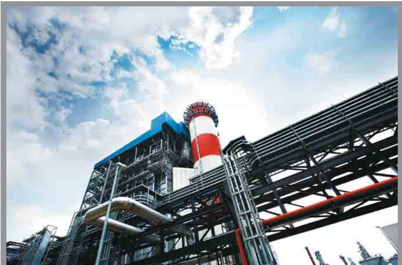
YTL PowerSeraya's Combined Cycle Co-Generation Plant at Jurong Island, Singapore
