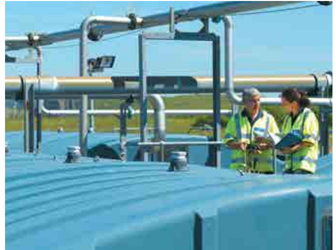
Reviewing energy efficiency at Wessex Water's Shaftesbury sewage treatment works in Dorset
