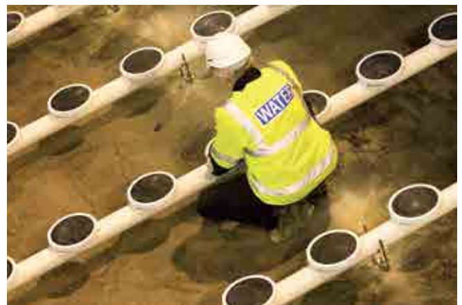
Upgrade of air delivery system at Weymouth Sewage Treatment Works to save energy
